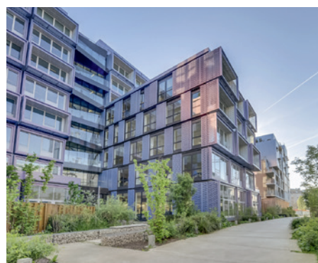
In Situ, Boulogne-Billancourt, France, office building
