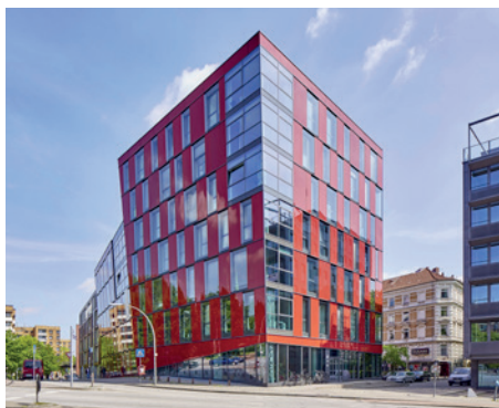
Dock 47, Hamburg, Germany, office building
