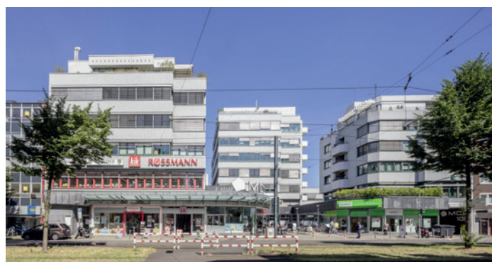
Münster Center, Düsseldorf, Germany, office, commercial and residential building
